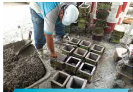
Construction waste is re-purposed into other useful products/materials at project sites
