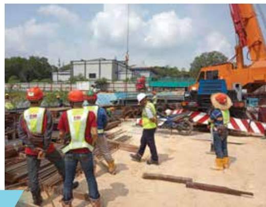
Safety training courses are conducted frequently to enhance awareness towards good health and safety practices at job sites
