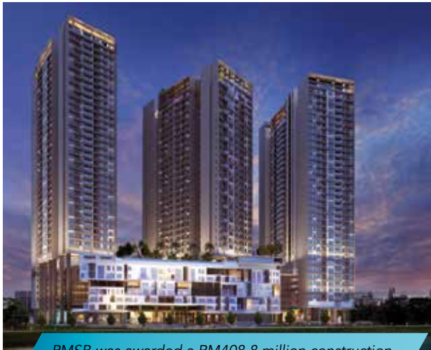
PMHB was awarded a RM408.8 million construction job for TRIA Seputeh Phase 2 by MRCB Builders in February 2019
