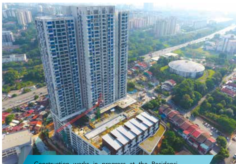
Construction works in progress at the Residensi Gen, Kuala Lumpur
