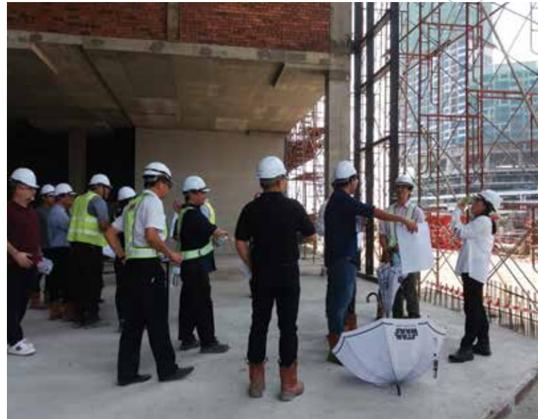
Site walk at Central Plaza i-City Mall with client
