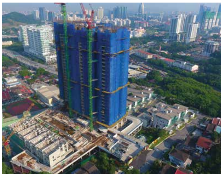
Work in progress at Residensi Gen, Kuala Lumpur
