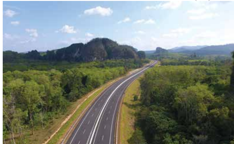
Central Spine Road, Segment 3E2 at Gua Musang, Pahang was completed in March 2018
