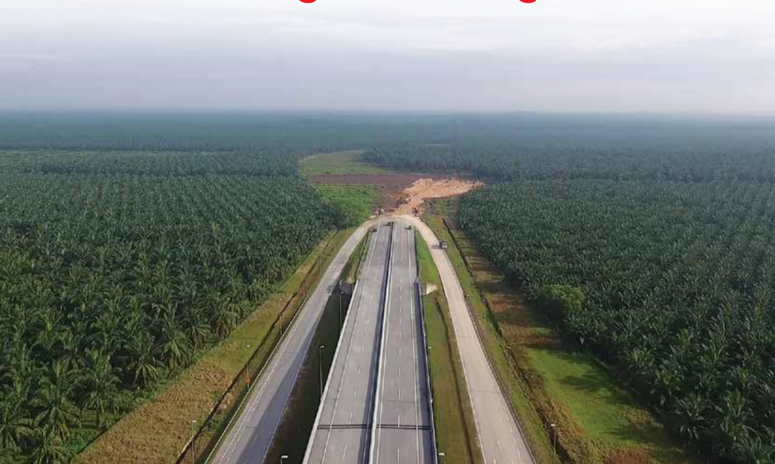
Work in progress at West Coast Expressway, Selangor
