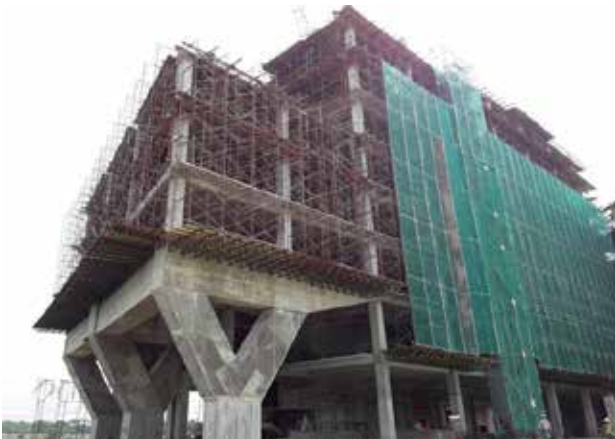
Y Columns at the KPJ Bandar Dato' Onn Specialist Hospital project
