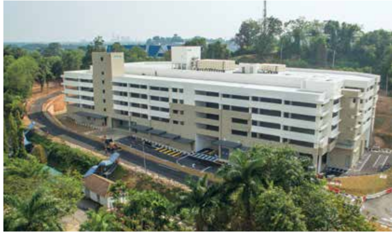
The Carpark Block for Pantai Ayer Keroh Hospital, Melaka was completed in March 2017
