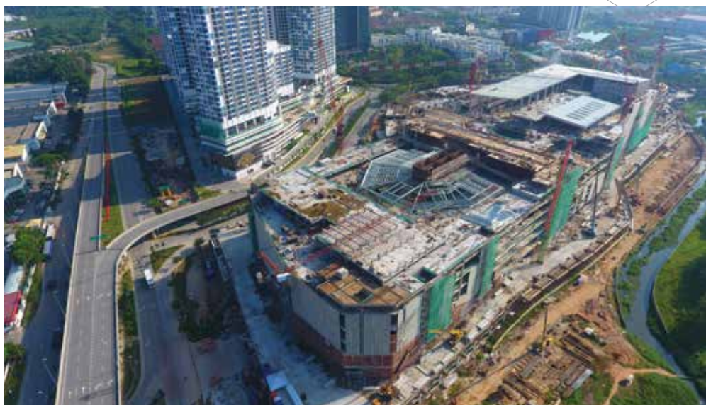
Work in progress at Central Plaza i-City Mall, Selangor
