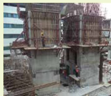
Normal Jump-form for lift core/ shaft
