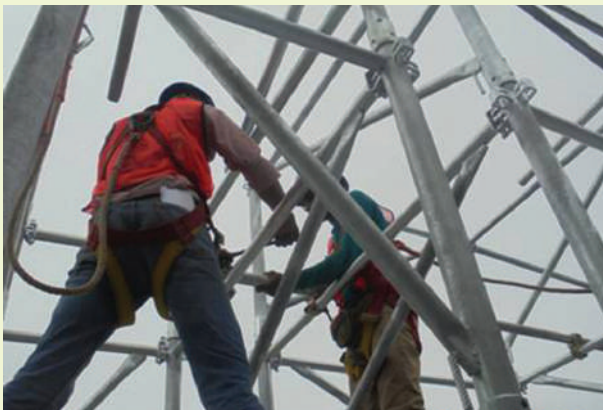
PPE compliance while working at height and top floor
