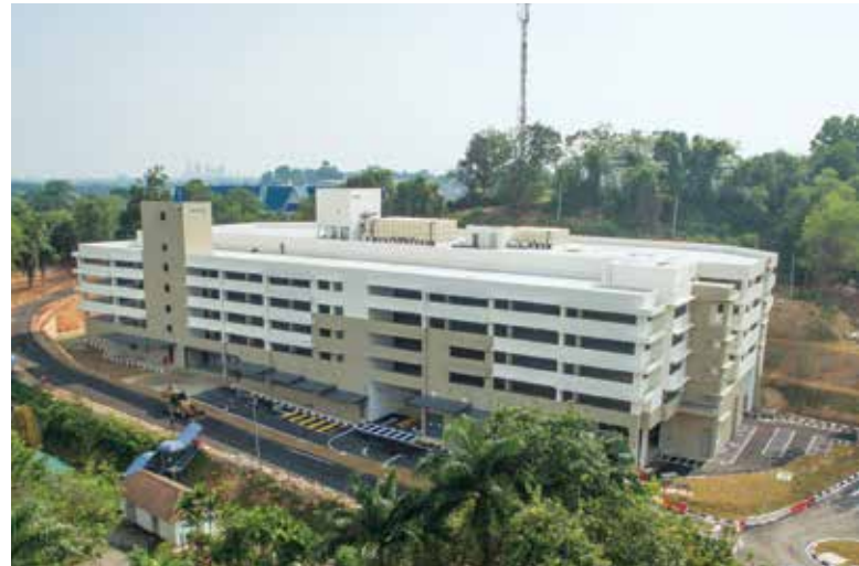
Carpark Block for Pantai Ayer Keroh Hospital, Melaka
