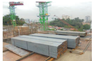
Proper materials arrangement according to the 5-S requirements to ensure the safety of all workers
