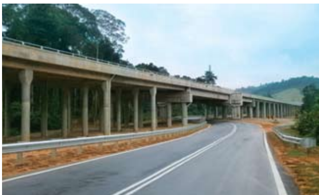
Gua Musang : Upgrading roadworks along Jalan Laluan 8 (Phase 1, Segment 5), Kelantan.
